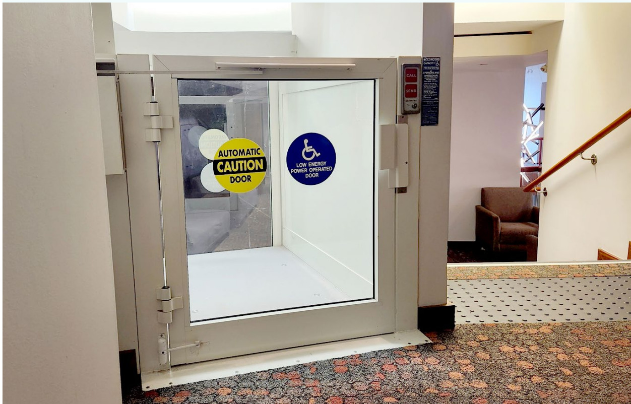
Image Description: The upper entrance to the secondary lift.
