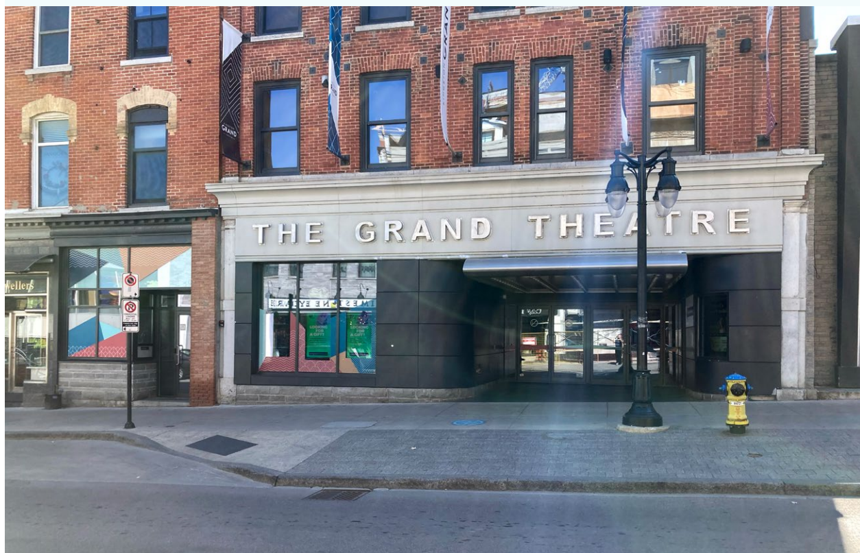
Image Description: The front of Kingston Grand Theatre. On the left of the photo is the drop off zone.
